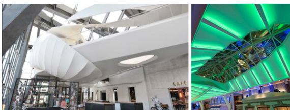
Fig. 12. Suspended PVC installations [23]
